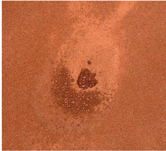
Damage to courts due to playing on wet courts
